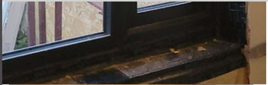
Air tight tape to window and from closer to brick Cill will have worktop to window. We will install some more insulation to it then
